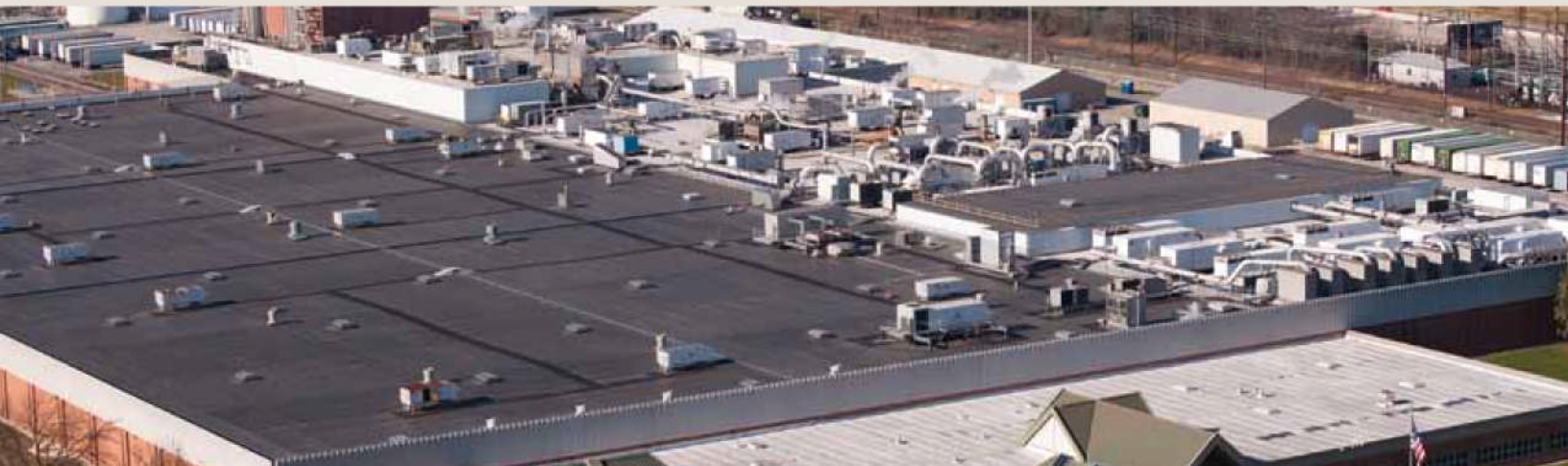
Kellogg Company Plant and Bakery - Lancaster, Pennsylvania
