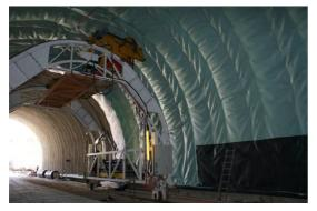
pneumatic test with air.
